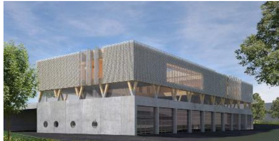
Fire Station, Straubenhardt, Germany
