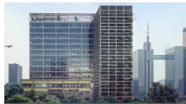
Renovation of WTC-Towers, Brussels, Belgium
