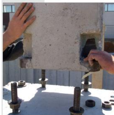
Photos showing the steps in the process of assembling the Peikko Column Shoes.
